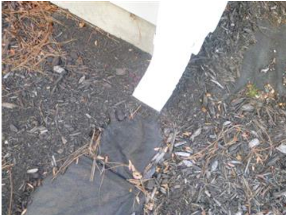
Washout Under Downspout
