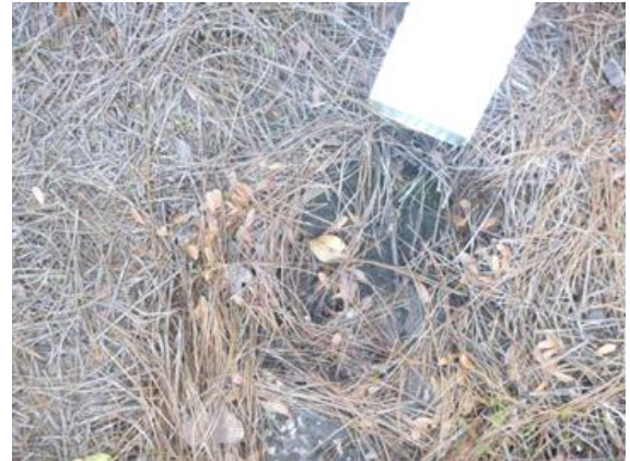
Depression Under Downspout
