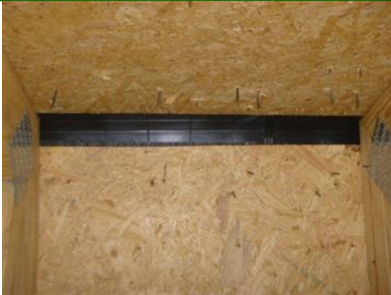
Interior Of Ridge Vent
