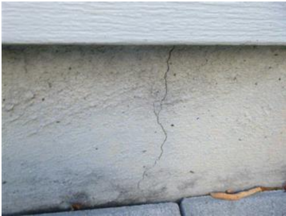
Left Side Crack
