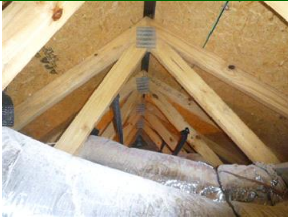
2" x 4" Truss Framing
