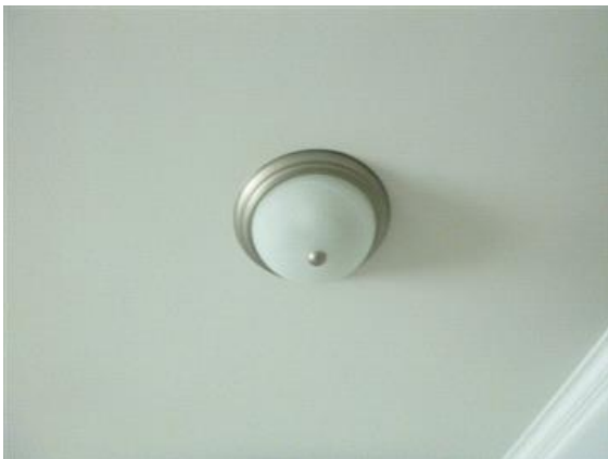
Ceiling Light Out
