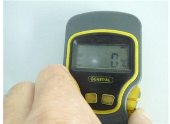
Normal Moisture Reading On And Around The Stain
