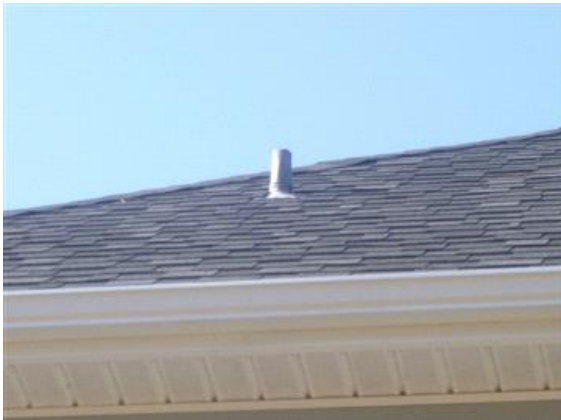
Typical Lead Plumbing Vent Flashing
