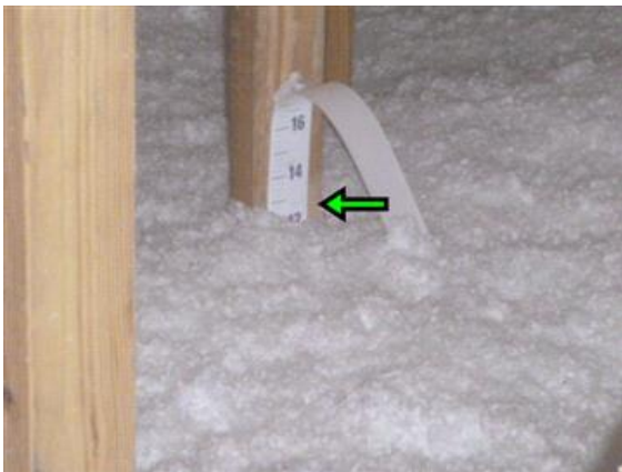
Loose Fill Insulation
