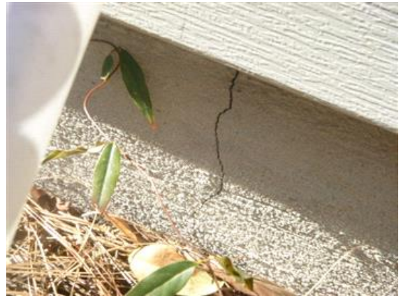
Left Side Crack
