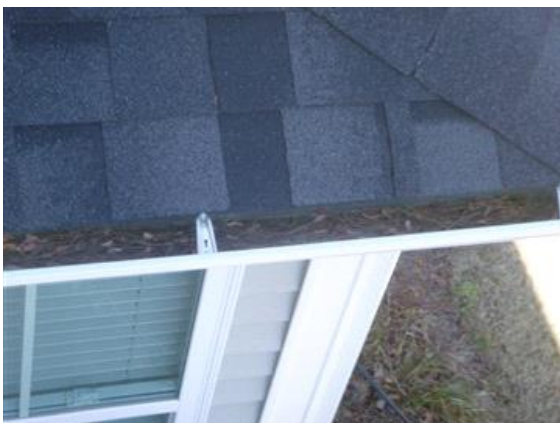
Debris In Gutter
