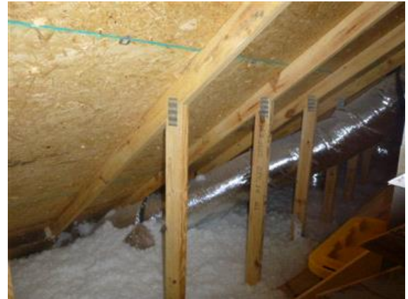
2" x 4" Truss Framing
