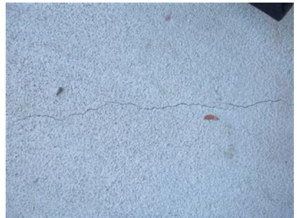
Crack Front Of Porch
