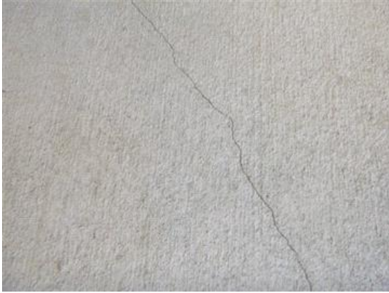
Crack Left Side Of Porch
