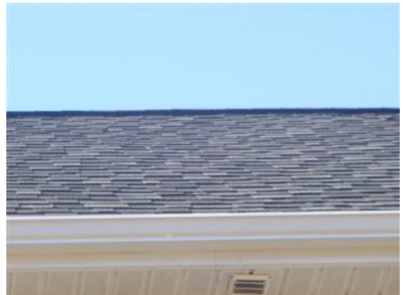
Exterior Of Ridge Vent
